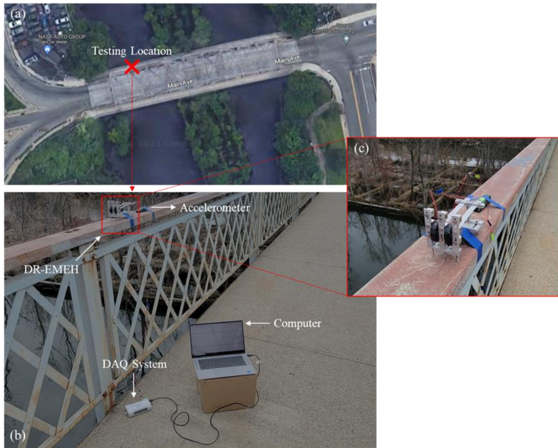
Figure 4.8. Field testing of the DR-EME on the Main Avenue Bridge in NJ: (a) photo of the bridge taken from the Google map with the location of testing marked, (b) testing setup, and (c) mounting of the device on the sidewalk railing.
