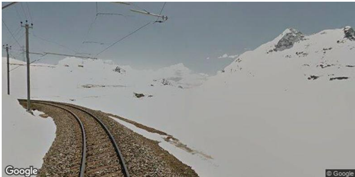
Figure 3-6 Sample Street View Image Captured by Google Static API
