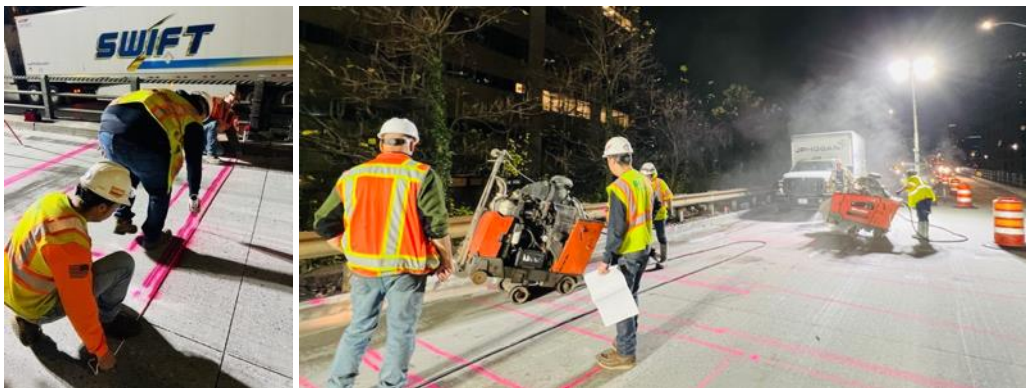
Figure 6: Marking sensor location and Sawcutting for Quartz sensor and loop
