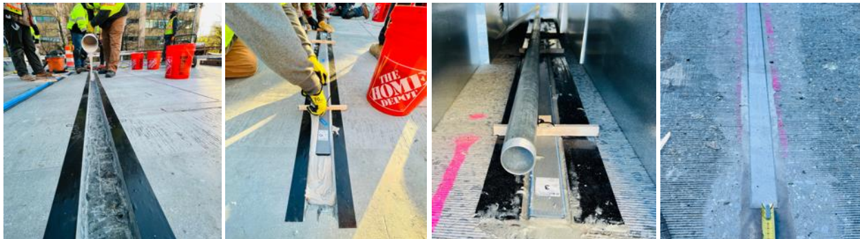
Figure 7: Sensor installation – Epoxying, Installing, Curing, and Grinding.
